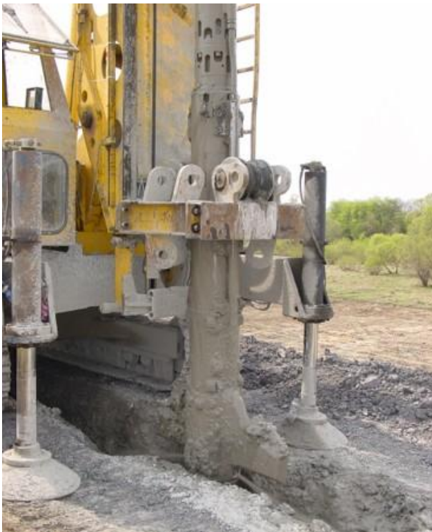
Fig. 11. Example of vibro method using wing vibrator (Gluszkiewicz, 2002).
