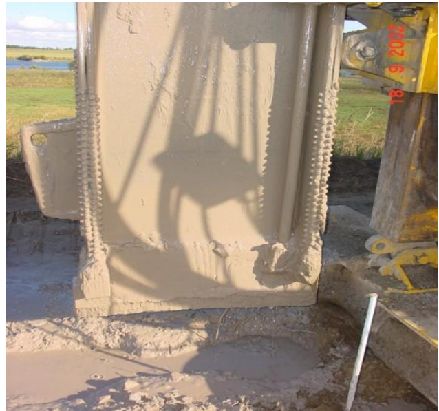
Fig. 12. Example of vibro method using hanged H-beam (Gluszkiewicz, 2002).
