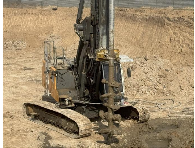
Fig. 6 Equipment for DSM technology – single mixing tool.
