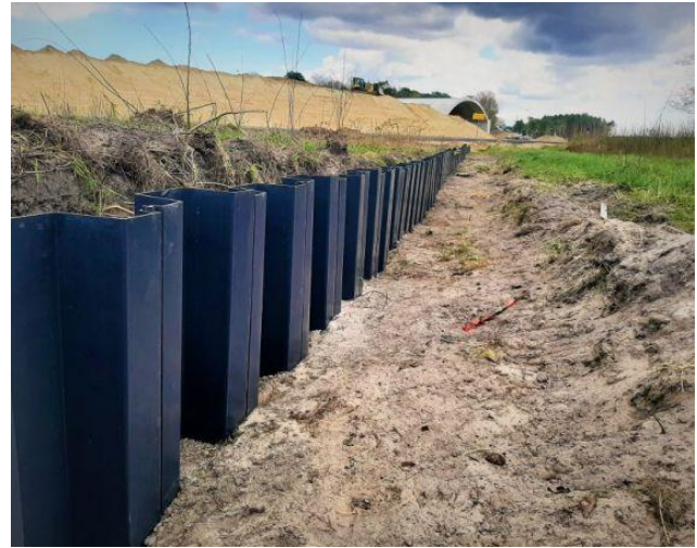
Fig. 10 Example of already installed vinyl sheet piles (10).
