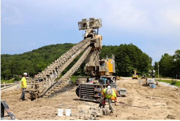
Fig. 4 Equipment for vertical trenching method (12).
